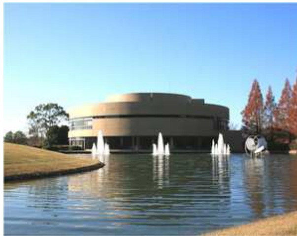
The main building of HARL
